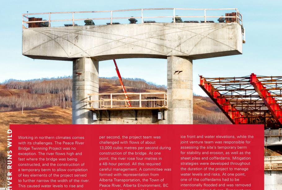
Working in northern climates comes with its challenges. The Peace River Bridge Twinning Project was no exception. The river flows high and fast where the bridge was being constructed, and the construction of a temporary berm to allow completion of key elements of the project served to further narrow the width of the river. This caused water levels to rise and the river to flow even faster. Although the river typically flows at an average rate of about 2,000 cubic metres
