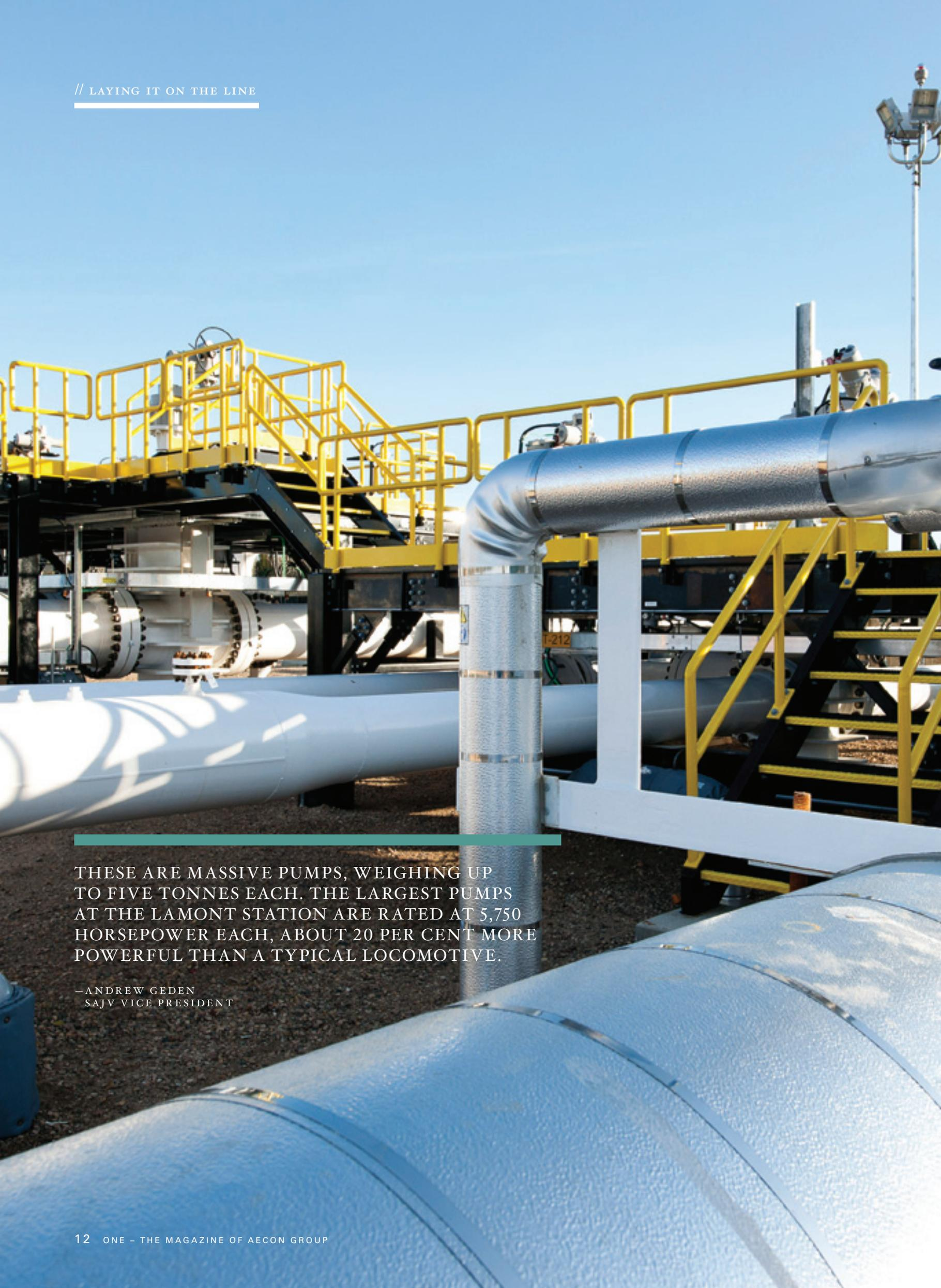
THESE ARE MASSIVE PUMPS, WEIGHING UP TO FIVE TONNES EACH. THE LARGEST PUMPS AT THE LAMONT STATION ARE RATED AT 5,750 HORSEPOWER EACH, ABOUT 20 PER CENT MORE POWERFUL THAN A TYPICAL LOCOMOTIVE.
