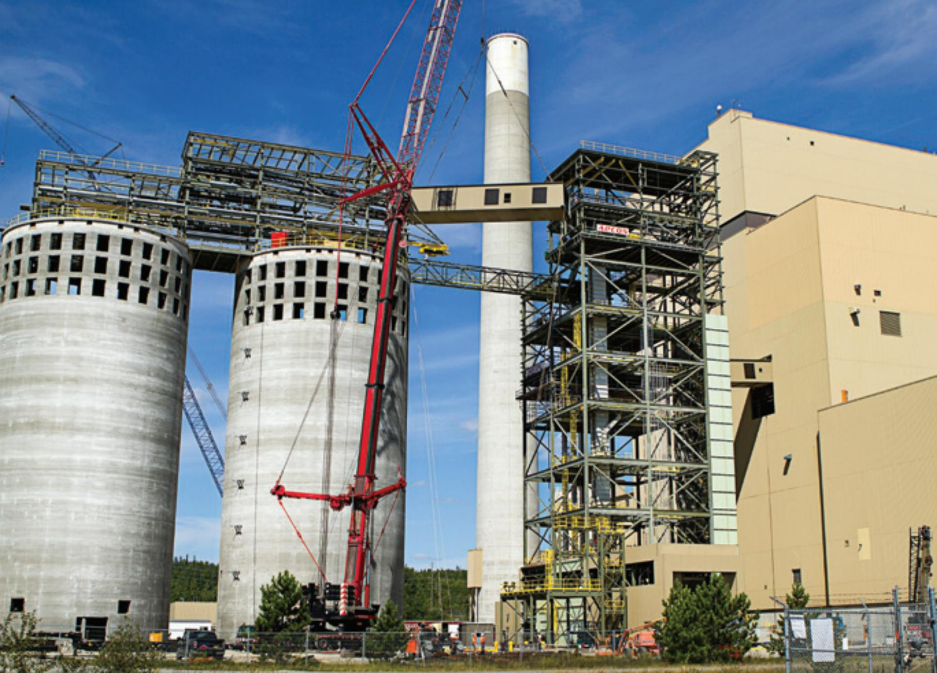
Conveyor bridges connect the mechanical rooms at the top of each silo and the transfer station to the power station. Each bridge was built as prefabricated modules with the wiring, lighting, ductwork, piping and cable trays installed before the bridge was lifted into place 50 metres above the ground by a 600-tonne crane.
