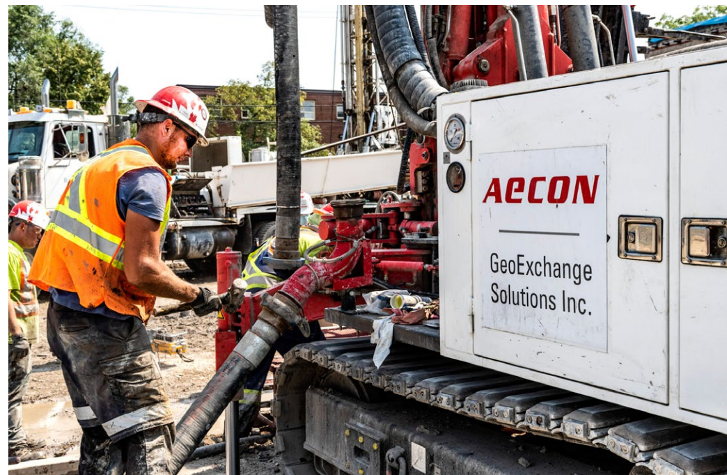
☑ Aecon employees installing a GeoExchange system
