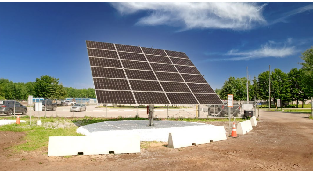
☑ Solar tracker installed at Aecon's Training and Innovation Centre in Holland Landing, Ontario
