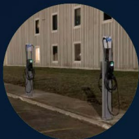
EV Charger Installations on Aecon Properties
