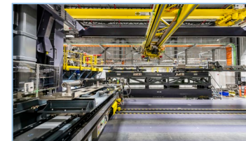
Bruce Power Fuel Channel and Feeder Replacement
