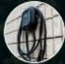
EV charger installation
