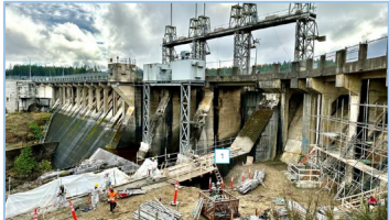
John Hart Dam Seismic Upgrade Project
