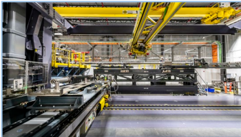
Bruce Power Fuel Channel and Feeder Replacement
