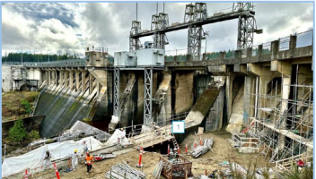
John Hart Dam Seismic Upgrade Project
