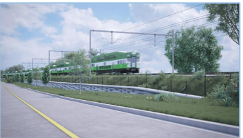
GO Rail Expansion On-Corridor Works
