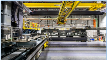
Bruce Power Fuel Channel and Feeder Replacement
