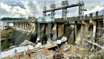
John Hart Dam Seismic Upgrade Project
