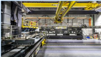
Bruce Power Fuel Channel and Feeder Replacement
