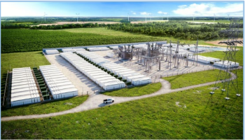
Oneida Energy Storage Project
