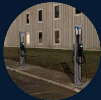
EV Charger Installations on Aecon Properties
