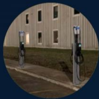
EV Charger Installations on Aecon Properties
