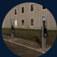
EV Charger Installations on Aecon Properties
