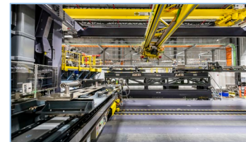
Bruce Power Fuel Channel and Feeder Replacement
