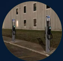
EV Charger Installations on Aecon Properties
