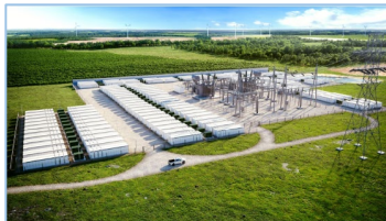
Oneida Energy Storage Project
