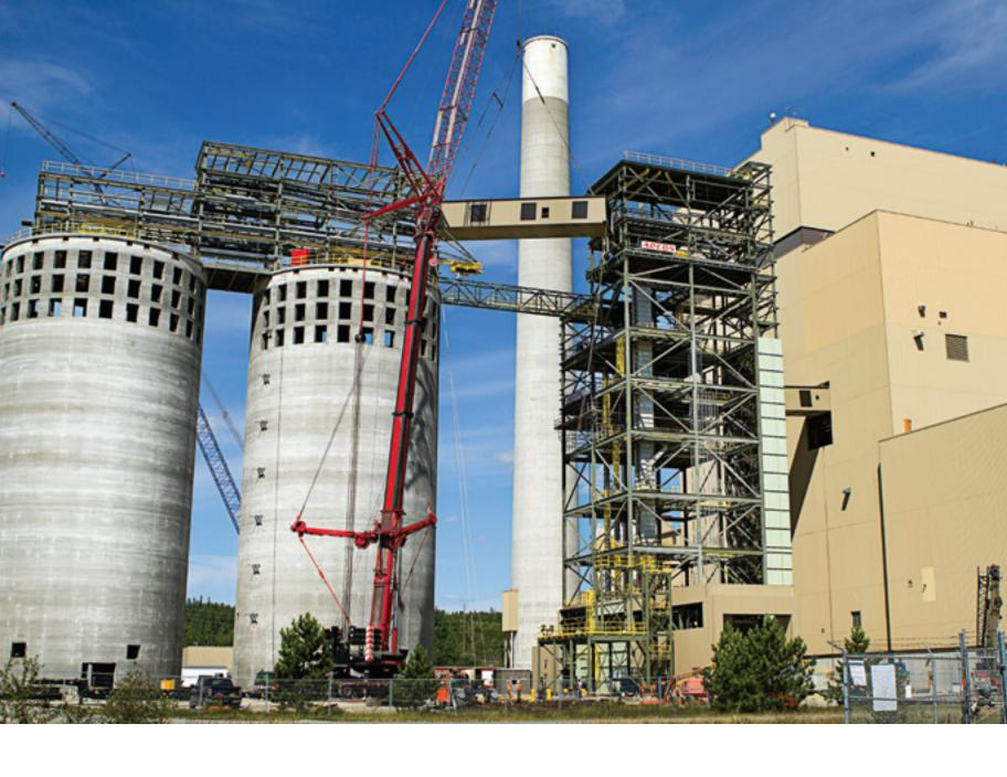
Conveyor bridges connect the mechanical rooms at the top of each silo and the transfer station to the power station. Each bridge was built as prefabricated modules with the wiring, lighting, ductwork, piping and cable trays installed before the bridge was lifted into place 50 metres above the ground by a 600-tonne crane.
