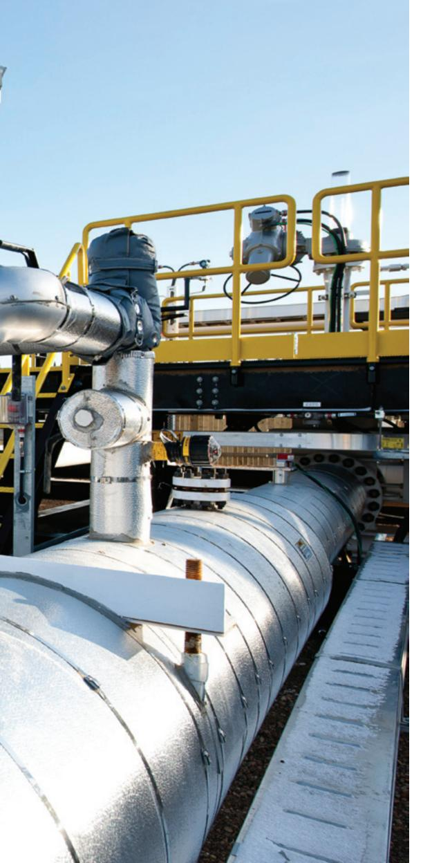
That means that our level has to be within 0.008 per cent." Once the pads are level, the crew sets a heavy steel base plate on top and, after a few fine adjustments, grouts the assembly into place. The pump and motor are then lifted into place and aligned with lasers, with steel shims used to make the final levelling adjustments. All in all, it takes about 10 days to level each plate and install the equipment, after which the crew completes the wiring and the piping.
