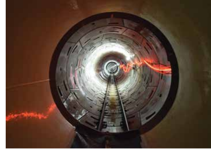
Pipe travelling within the tunnel
