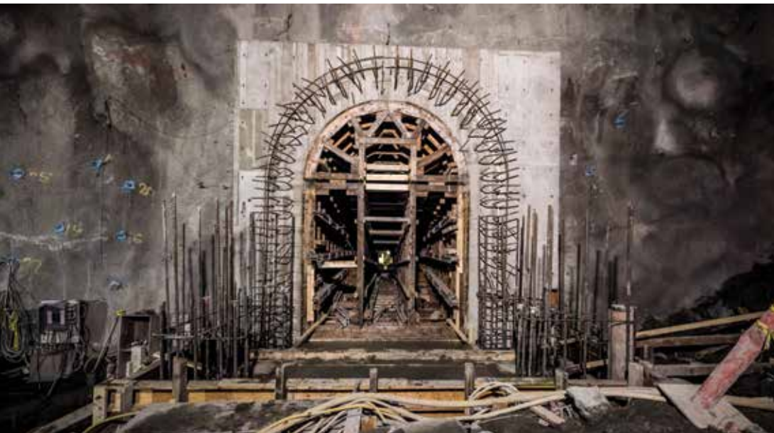
One of the turbine/generator outlets leading into the surge chamber
