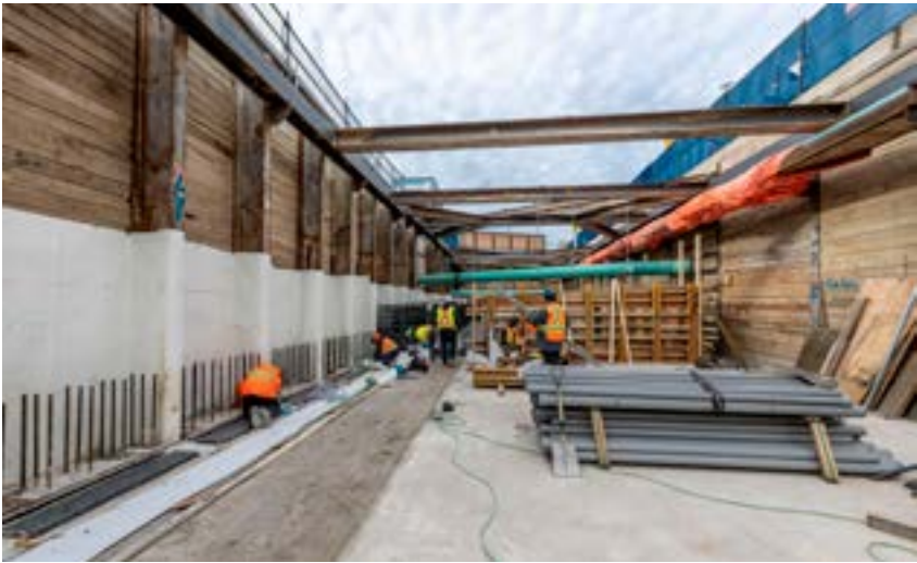
Open cut excavation at Fairbank Station
