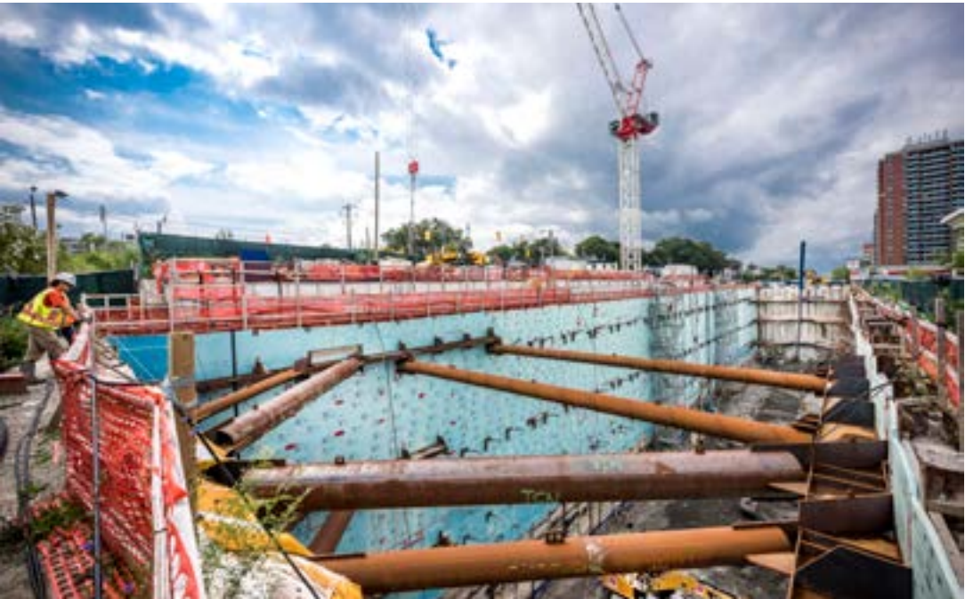
Open cut excavation at Caledonia Station
