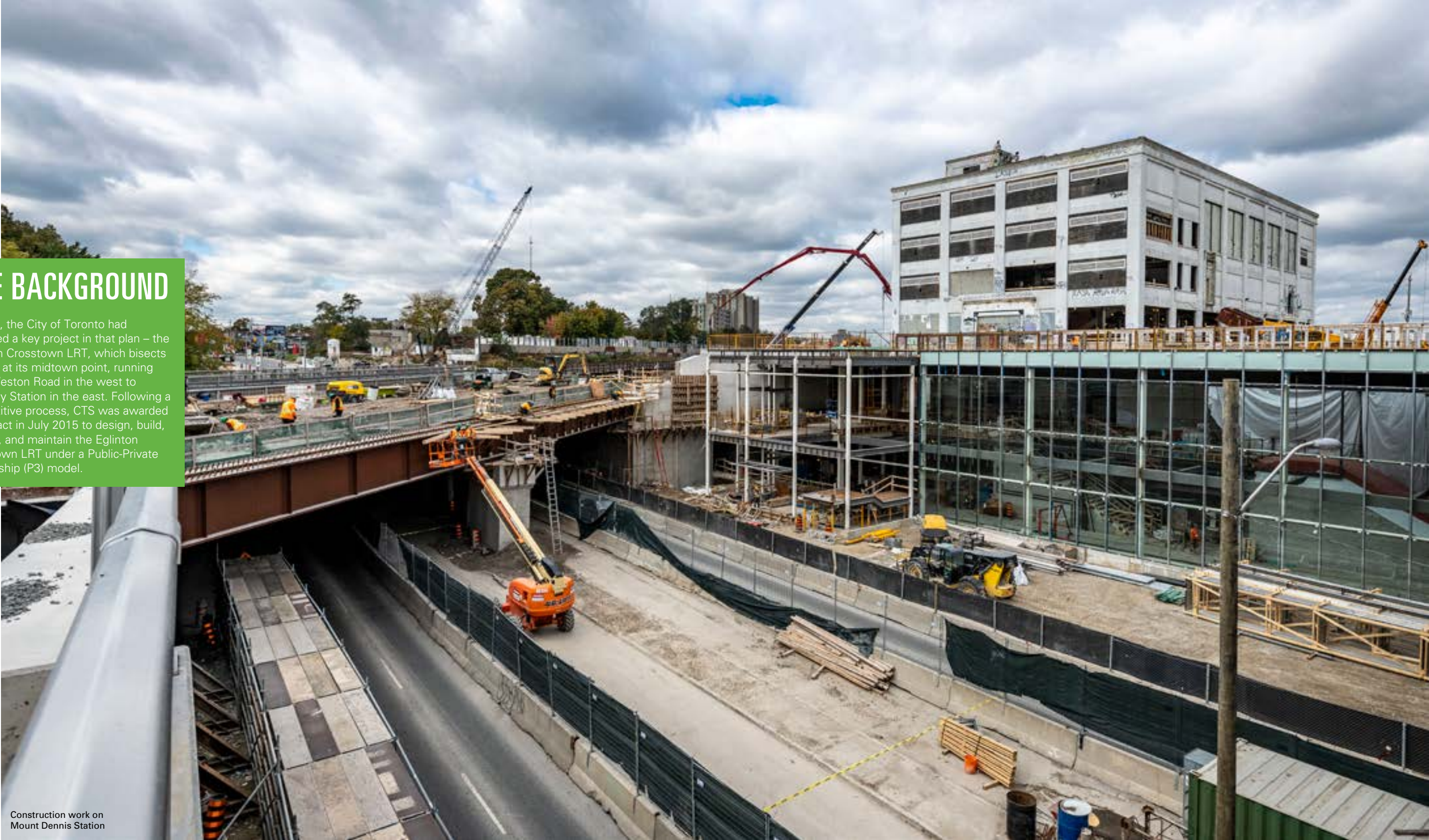
Open cut excavation at Fairbank Station
