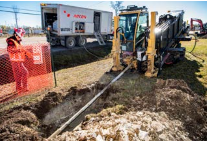
One of two new specialized horizontal directional drills on the job
