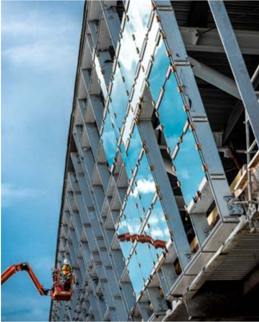
A worker installs the exterior envelope of the new terminal
